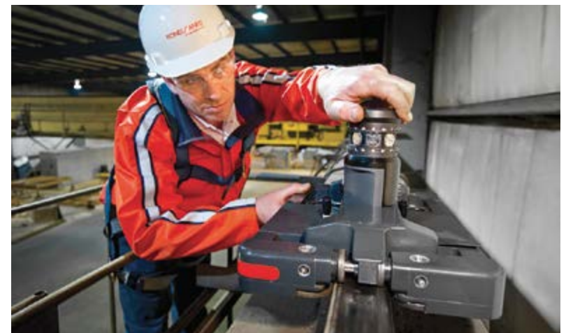
RailQ reduces runway surveying time from days to hours.
