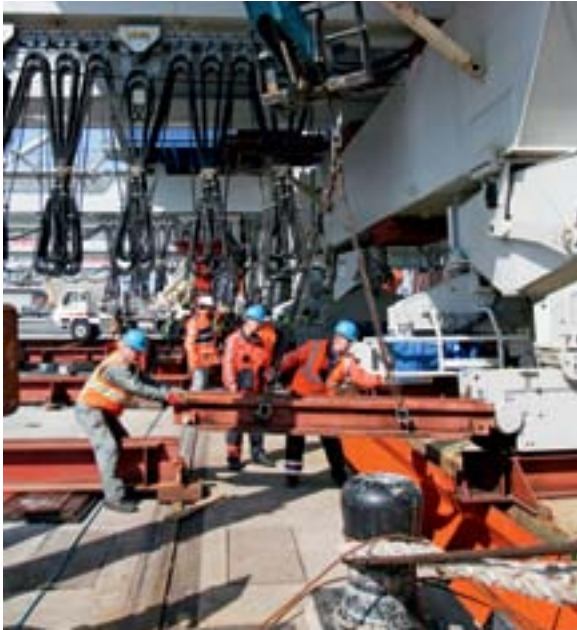
Getting the cranes out of the ship is challenging and complicated.
